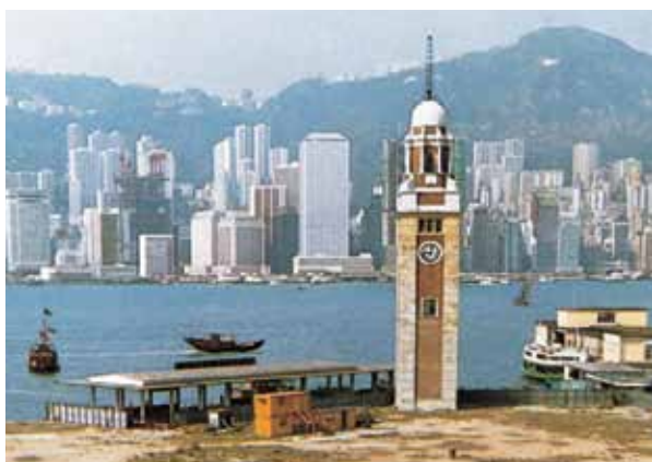
The Kowloon-Canton Railway clock tower has seen Hong Kong develop from colonial outpost to bustling metropolis.
